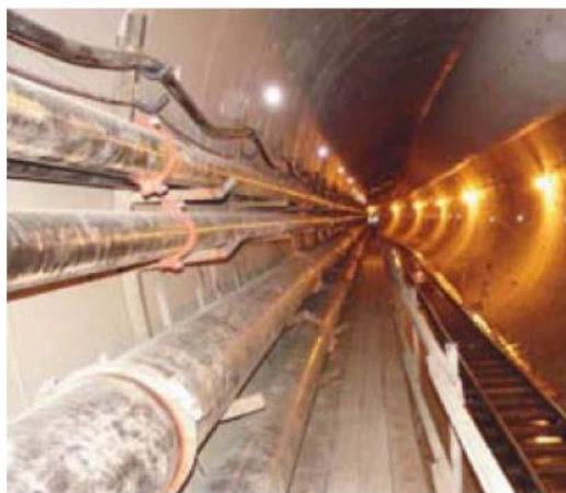
14" and 16" R-88 couplings used at the Eastside Combined Sewer Overflow Tunnel Boring Project – Portland, Oregon, USA.
